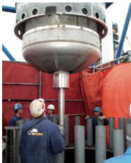
▲ Installation ammonia converter basket
