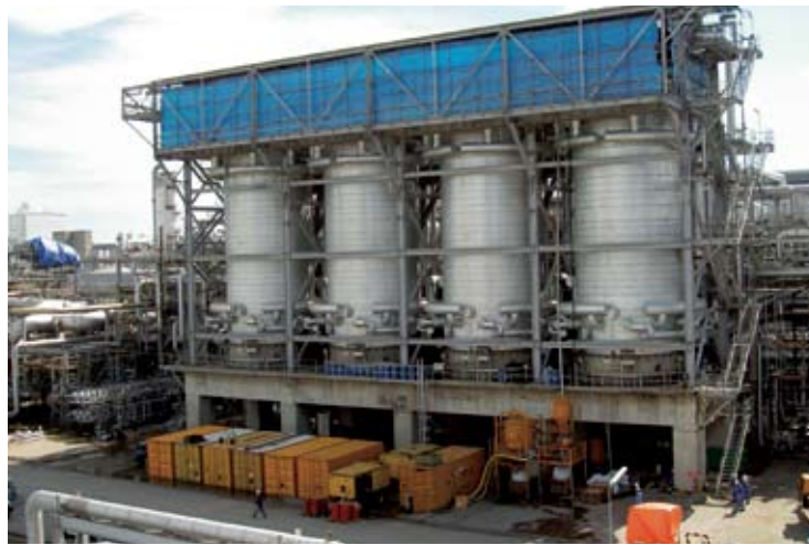
▲ Tubular reactor catalyst change out area
