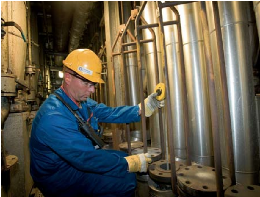
▲ Measuring the outage of a reformer tube
