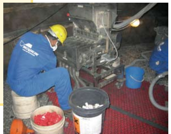
▲ Progress control using coloured caps
