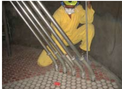
▲ Loading the catalyst by telescopic tubes
