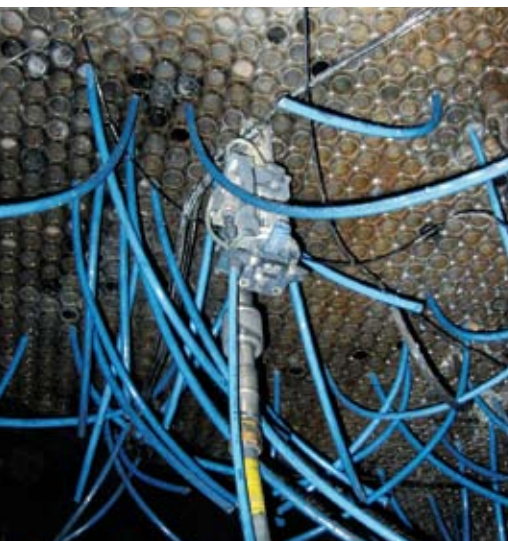
▲ TLE lance fixed to bottom of tube sheet
