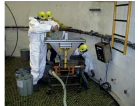
▲ Loading pre-bagged catalyst
