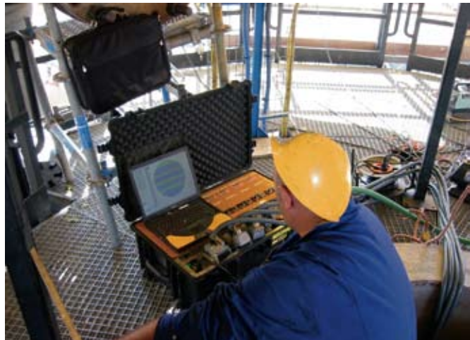
▲ Monitoring the progress of Pd measuring
