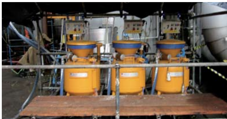
▲ Grit blast equipment set-up
