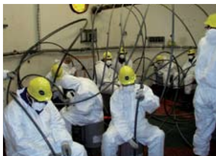
▲ Catalyst removal via direct vacuuming
