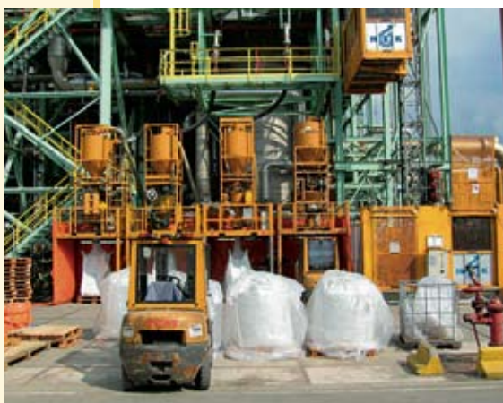
▲ Installing gas caps
