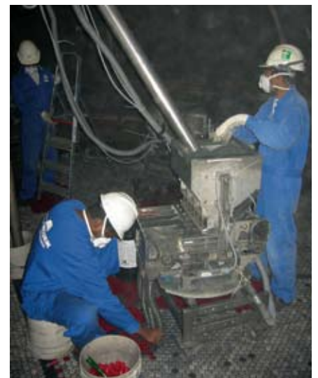
▲ Loading catalyst around the clock
