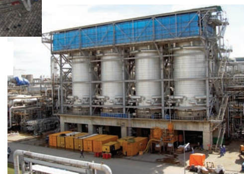
A tubular catalyst handling work area.
